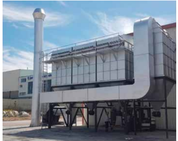
Exhaust gas filtration systems. Equipment example from ALM Company
